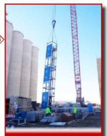
Angle frame slip tower typically sets in place with a crane in as little as one day.
